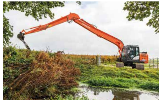
Special application excavators
